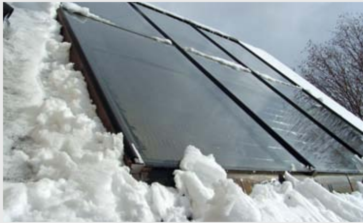
Stressing of the PV module
